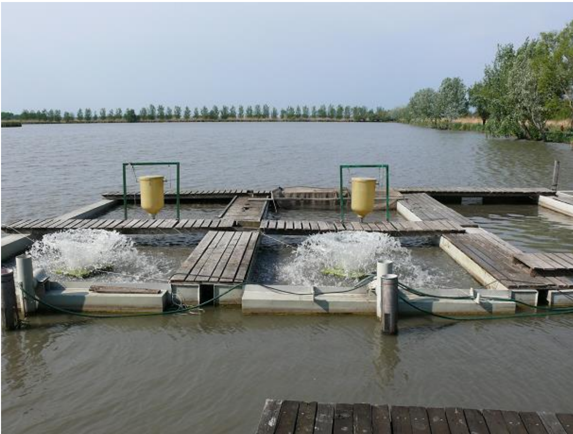
Figure 3 – "Pond-in-pond" system in operation in the fish farm of the "Jaszkiseri "Halas" Kft"
